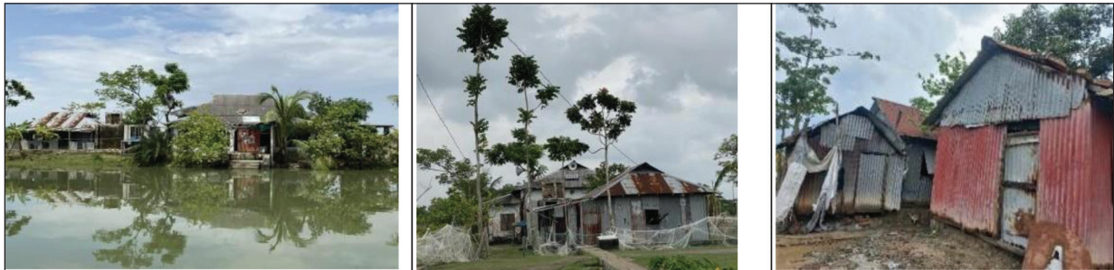
Figure 4: Site Surrounding, ORCA Palli: Water-Adjacent Homestead with Tin Roof and Vegetation Reflection (left); Cluster of Rural Dwellings Surrounded by Tall Palms and Open Path (middle); Dilapidated Corrugated Iron Houses with Visible Structural Damage (Right)
