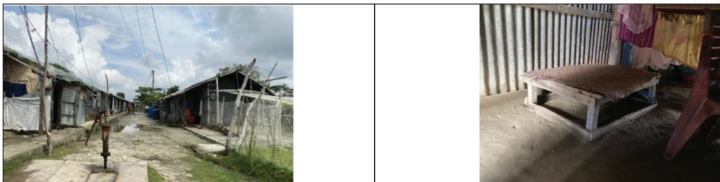
Figure 6: Existing Housing ORCA Palli 6: Narrow Lane Between Back-to-Back Houses with Overhead Wires (left); Interior Scene Showing Raised Bamboo Platform (Chouki) Over Mud Floor (right)
