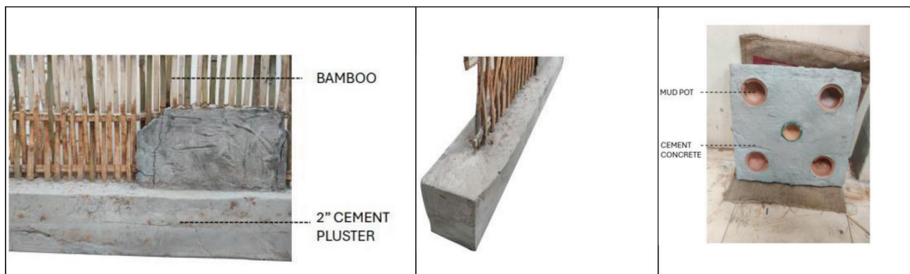
Figure 33: Bamboo & Cement Plaster (For Outer Walls), Mud Pot & Cement Concrete
