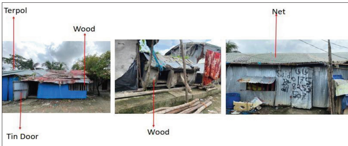
Figure 5: Existing Housing ORCA Palli 6: Tin and Roof with Bright Blue Walls and Tin Door (left); Makeshift Housing Structure with Wooden Framework and Temporary Coverings (middle); Corrugated Sheet House with Fishing Net Used as Faccade Screen (Right)
